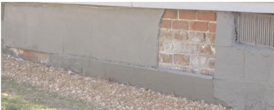
Moisture problems can cause paint failure on masonry (top) and block the adhesion of secondary coatings such as the parging seen here.
