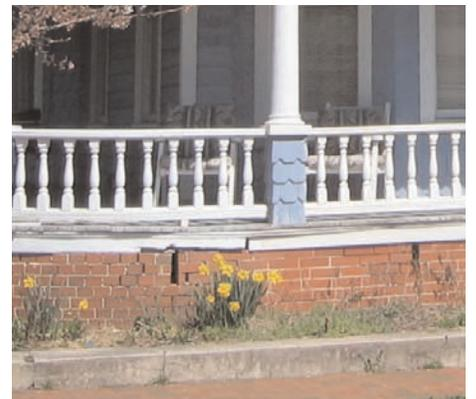
**i** Most foundations in Smithfield are of masonry. Brick piers are the most common and distinctive foundation type, especially for vernacular frame houses; many have been filled in with solid brick or concrete block; a few houses have stone foundations.
